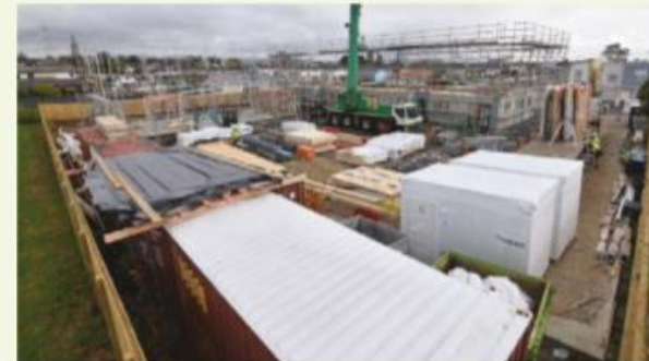
Progress at Busby Street on 3 June 2020, 18 of June then 26 of June.
